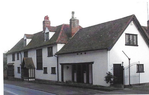
The leaded paned windows and deep porch are features of this property.
