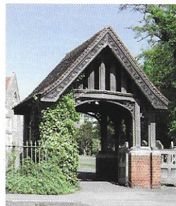
The Lych-gate leading onto Park Lane.
