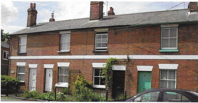
Red brick pre-war terrace York Road
