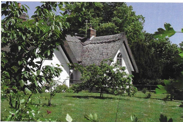
Thatched Cottages at the junction of Station Road.
