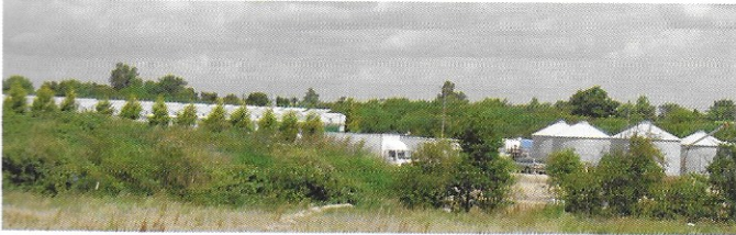
Glasshouses and Grain Stores at Hayhouse Farm.
