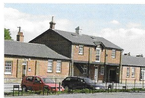
New businesses in the refurbished Atlas Works.
