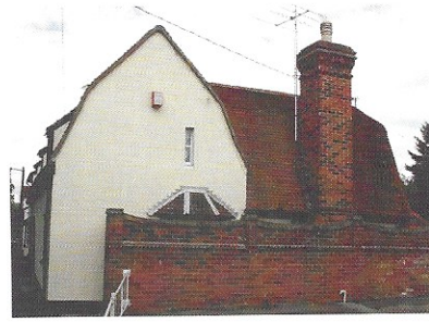
Side view of a Cottage in Lower Holt Street, illustrating a mansard roof, peg tiles and tall brick chimney. -
